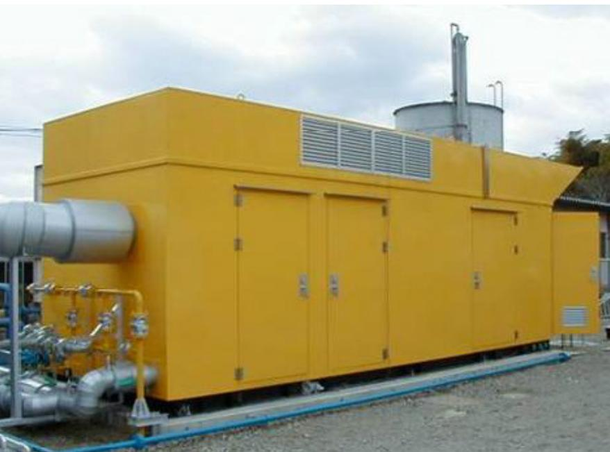
Figure 1: Typical Generator engine enclosure located adjacent to a customer site (Ref: Jenbacher)
